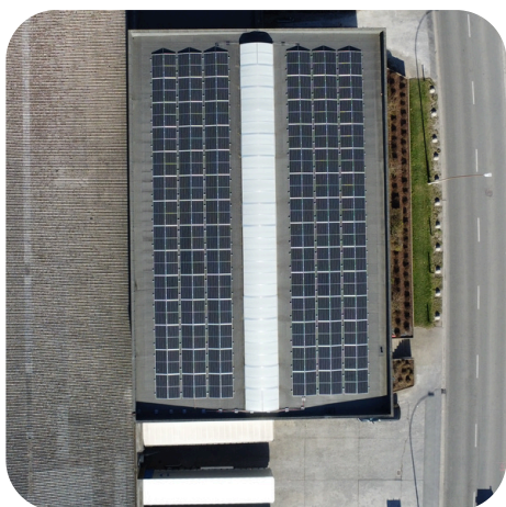
Plastuni Operations photovoltaic park
