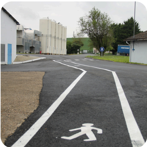
Redefinition of pedestrian walkways – Somater Marolles plant
